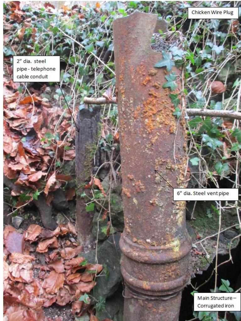
Fig 14 – Main entrance showing Ventilation and telephone cable pipes.
