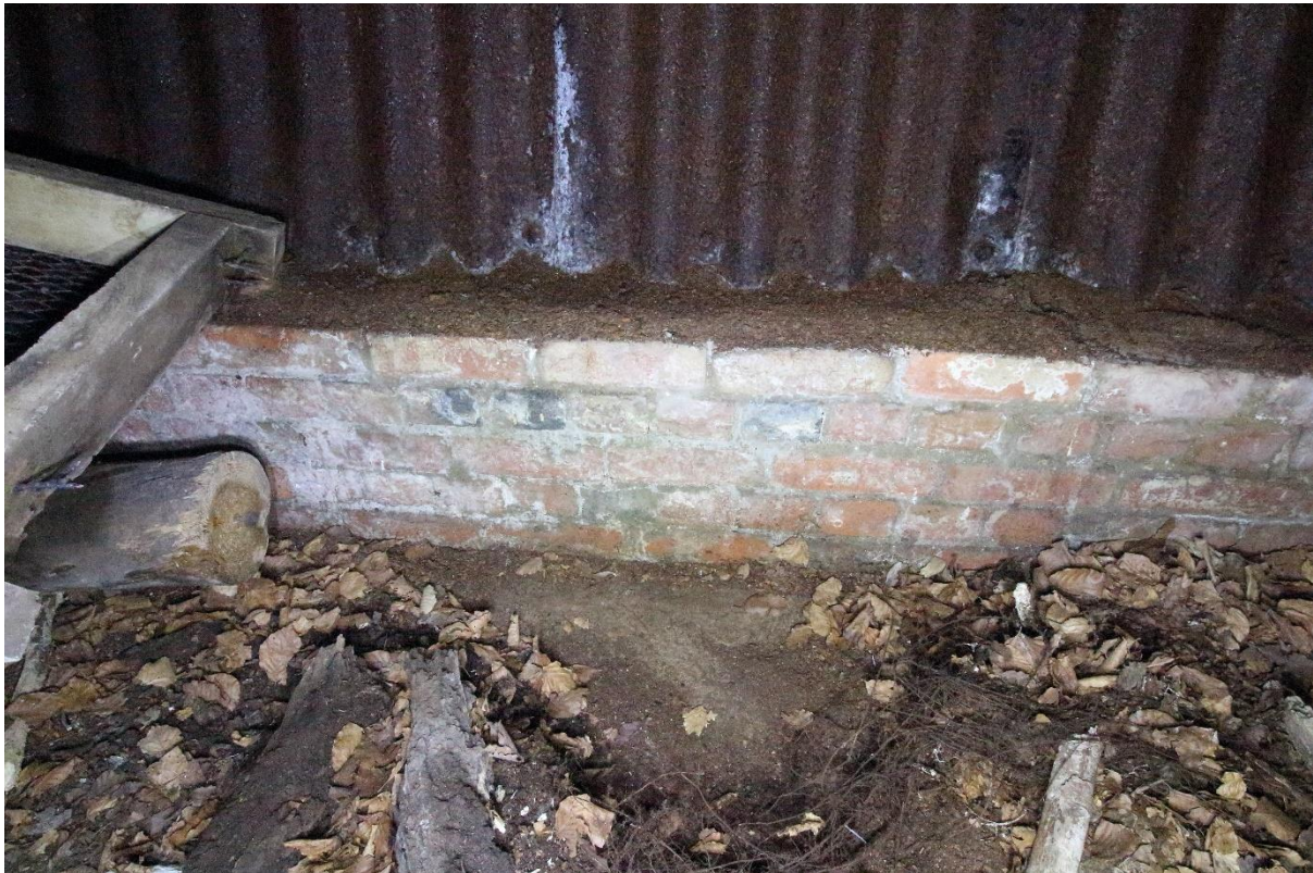
Fig 11 Concrete floor supporting 5 course brick walls and corrugated iron roof
