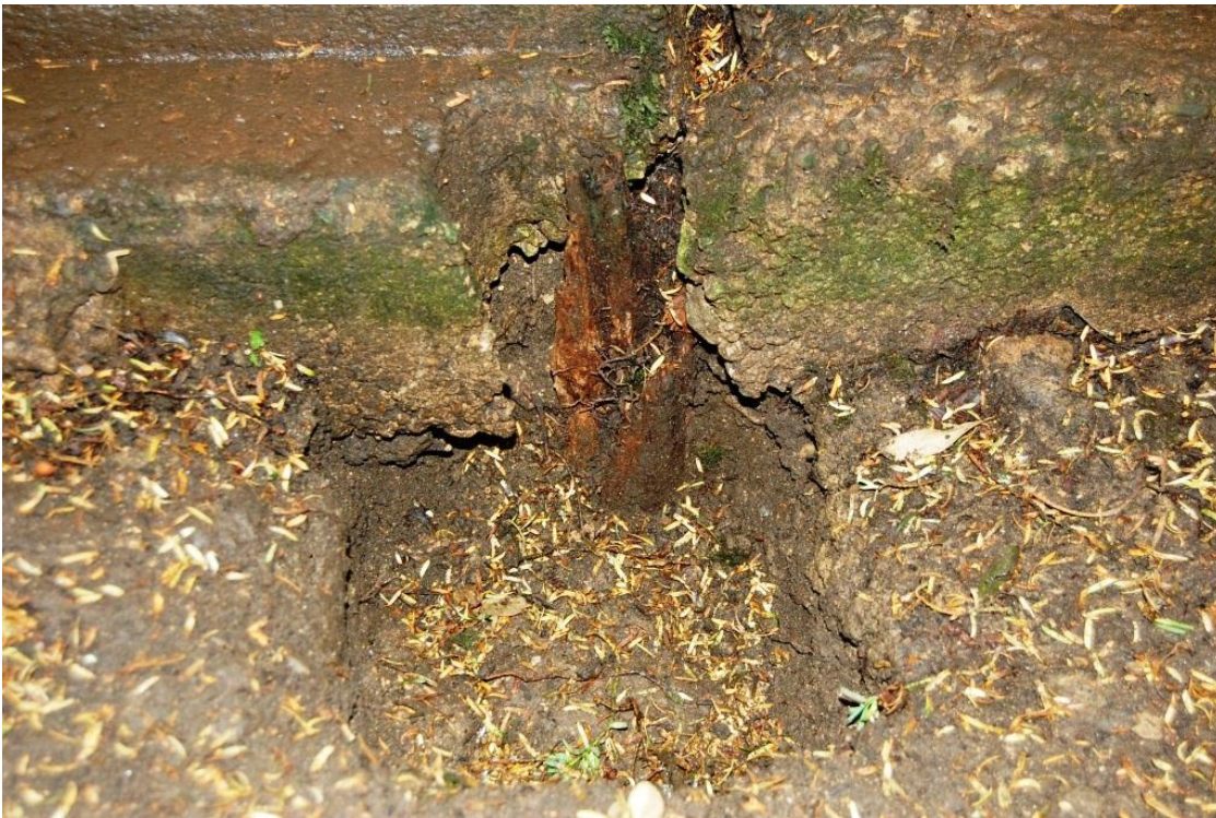
Photo 12: Structure 10 - Wooden stake in-situ (Photo No. CH07-11-0081)
